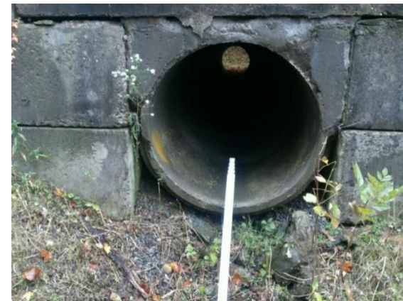
Fiddler's Bridge Rd
