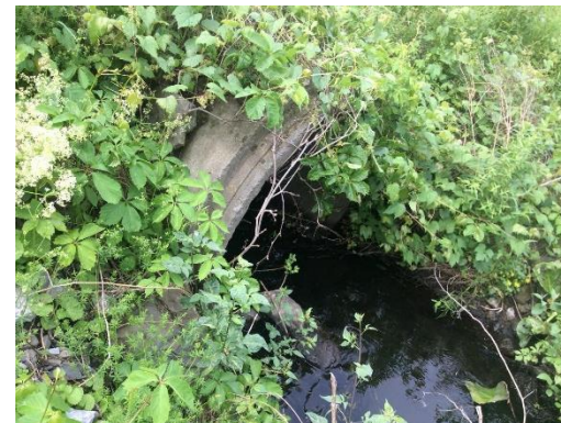
Fiddler's Bridge Rd
